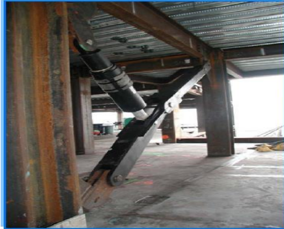
Viscous damper in a frame structure
