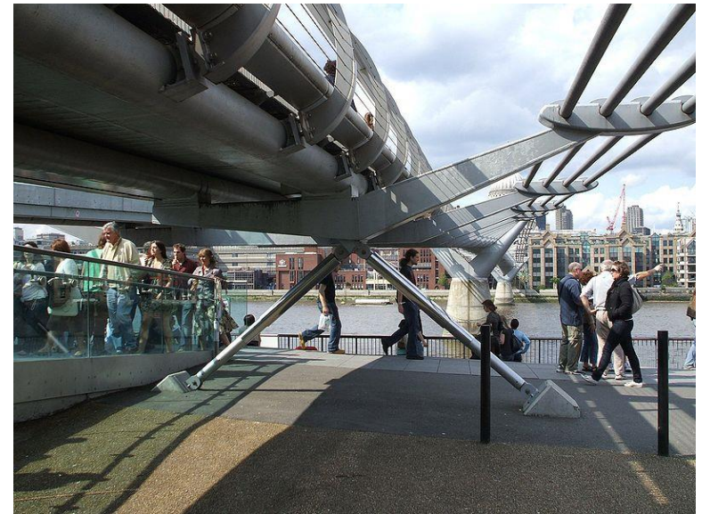
Viscous dampers for the Millennium bridge in London
