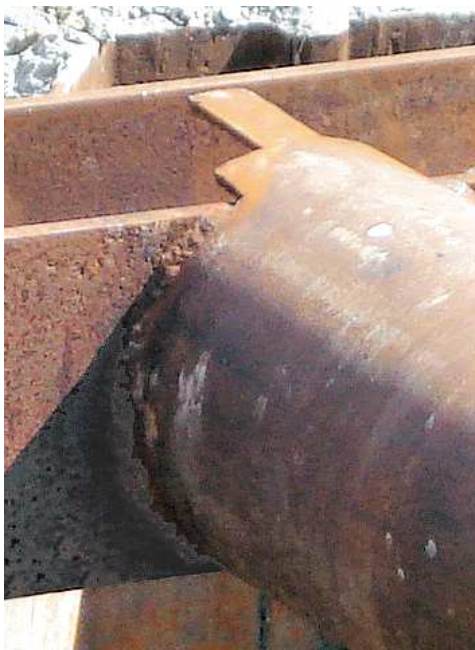
Figure 30-3 Welded connection of pipe strut and waling. The picture on the left (cofferdam near Sebastiaansbrug in Delft, 2007) shows a wale consisting of single H-profile, whereas the drawing on the right depicts the more common case of a double profile.
