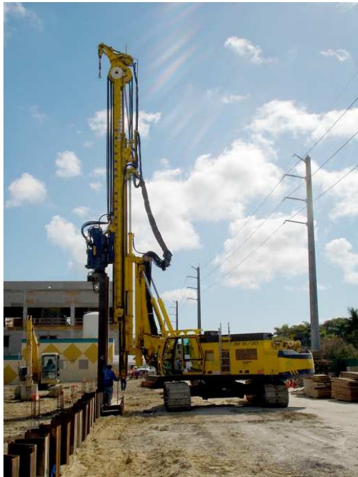
Figure 37-2 Driving a sheet pile ( http://www.hjfoundation.com/Services/Sheet-Piling/ )
