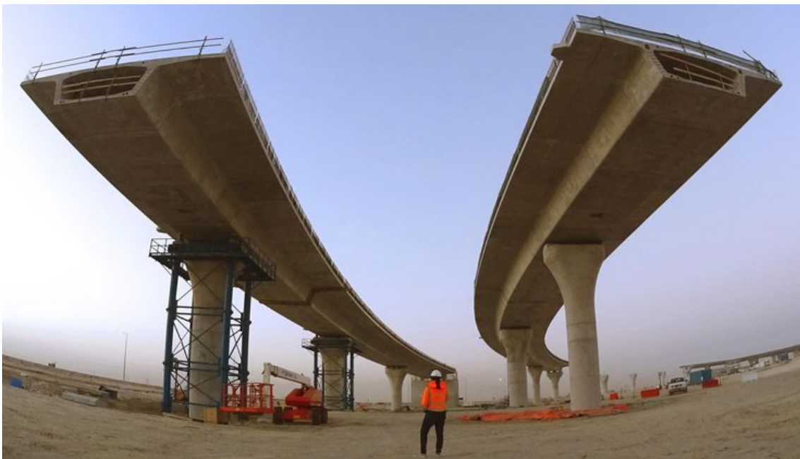
Fig 11.17 Box girders under construction (Doha, Qatar)
