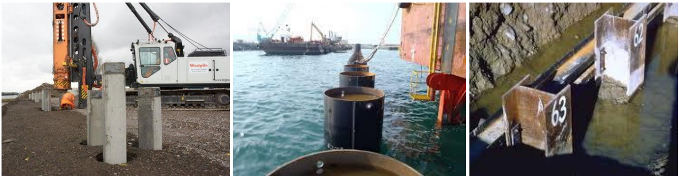
Figure 2.1 (a) Precast concrete piles, (b) steel open-ended tube piles and (c) Steel H-Piles
