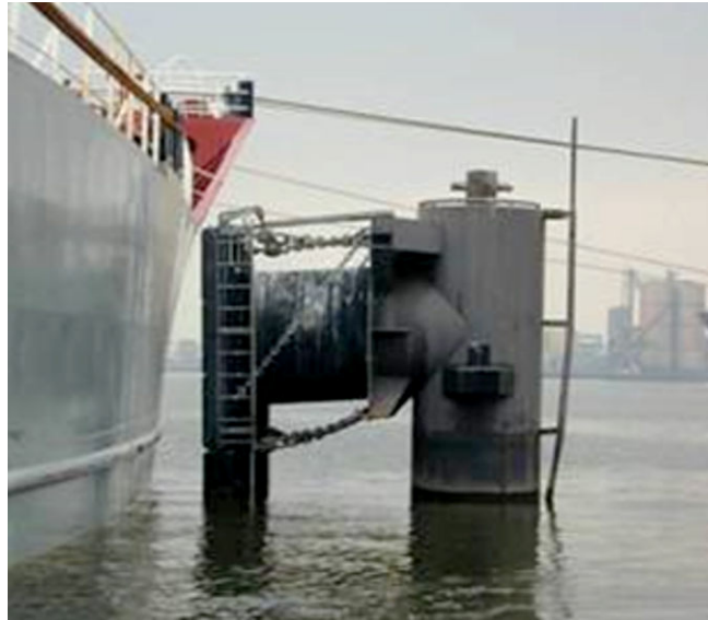
Figure 1.19: Flexible dolphin in the Port of Rotterdam
