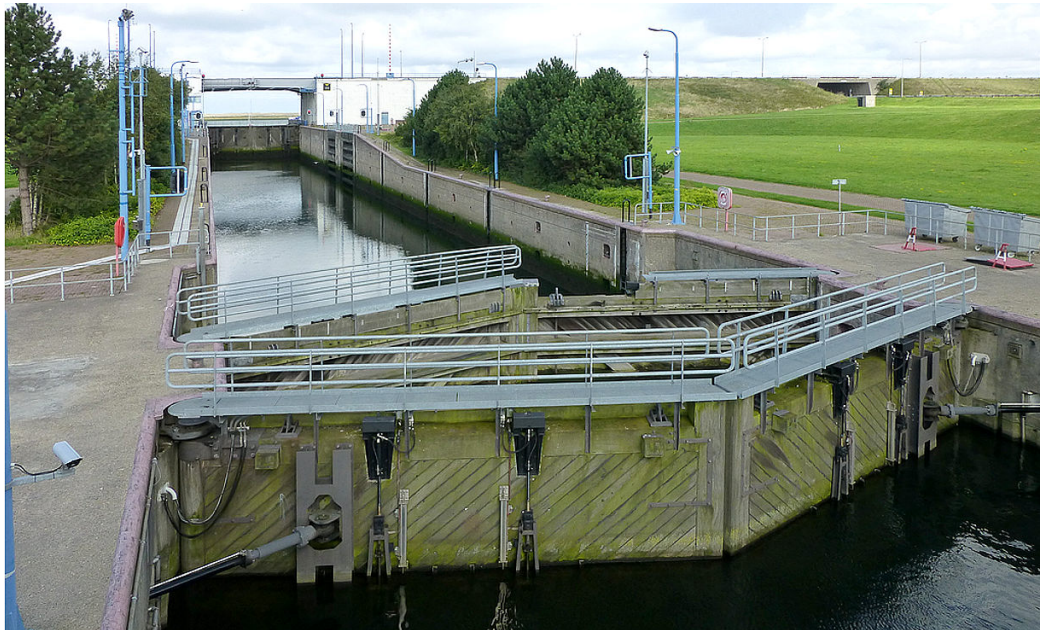
Figure 1.2: Navigation lock with mitre gates in the Haringvlietdam (TU Delft, 2014)
