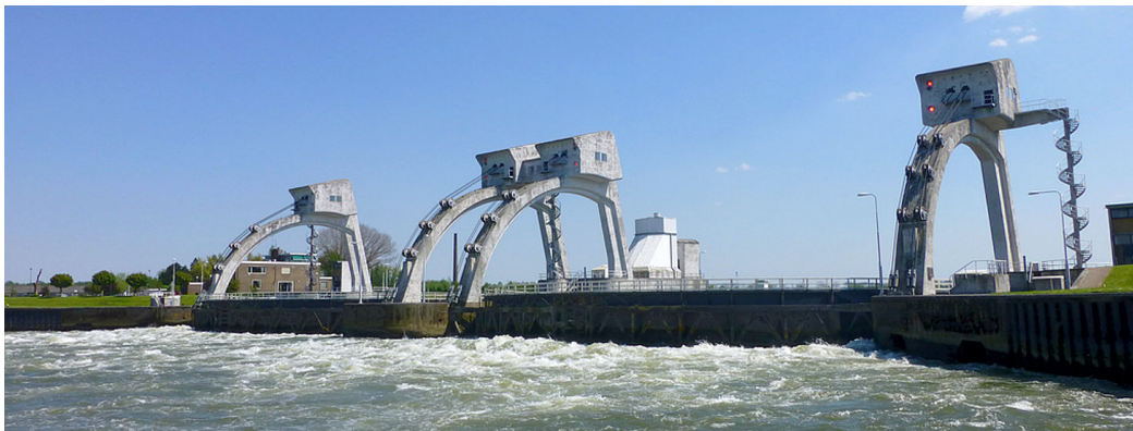
Figure 1.8: Visor weir in the Lek near Hagestein (TU Delft, 2016)
