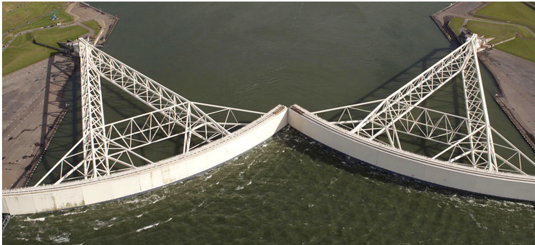
Figure 1.28: Storm-surge barrier in the Nieuwe Waterweg (Maeslantkering) (RWS)
