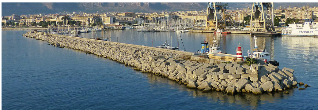
Figure 1.24: Breakwater in Palermo, Italy (TU Delft, 2015)
