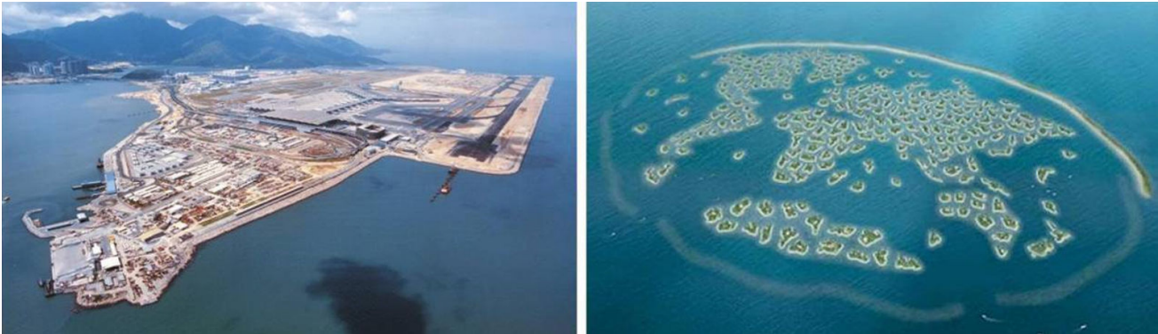
Figure 1.66: Artificial islands: Chek Lap Kok near Hong Kong (left) – World at Dubai (right) (sources unknown)
