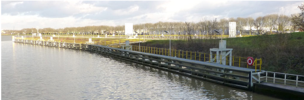
Figure 1.21: Approach wall near the navigation lock of Born (TU Delft, 2014)
