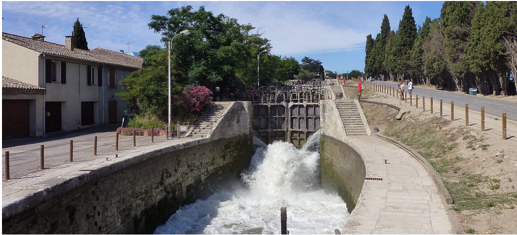
Figure 1.3: Staircase locks of Fonserannes in the Canal du Midi, France (TU Delft, 2015)
