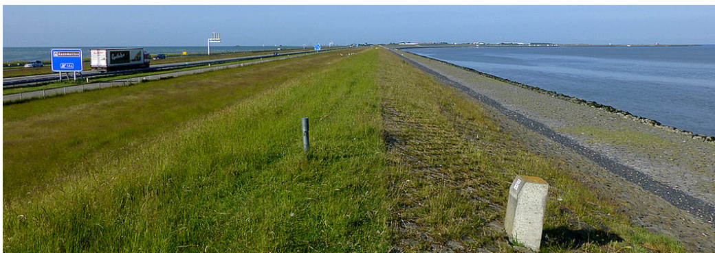
Figure 1.27: The 'Afsluitdijk', a closure dam, closing-off the IJsselmeer (TU Delft, 2014)
