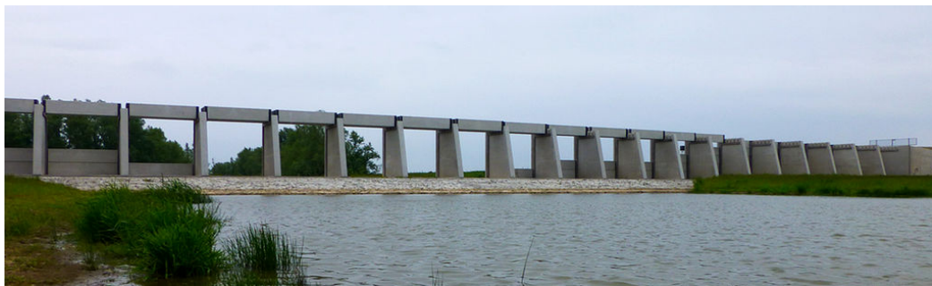
Figure 1.31: River discharge control structure near Pannerden (TU Delft, 2015)
