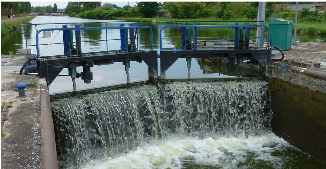
Figure 1.4: Gates of a lock can be used to regulate the water level in the upper canal section. Cambrai, France (TU Delft, 2015)
