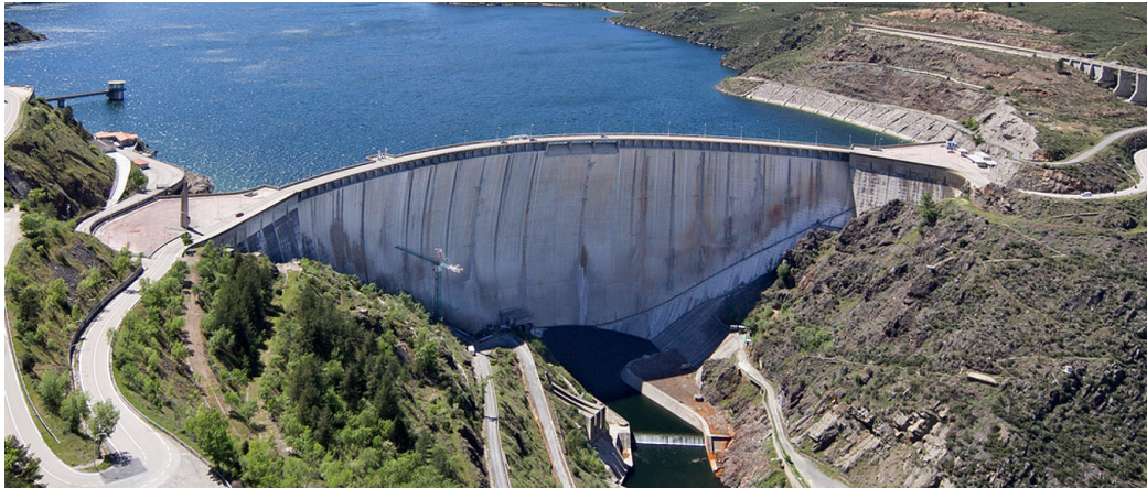
Figure 1.37: 'El Atazar' Concrete arch dam near Madrid, Spain (Wikimedia Commons, 2014)
