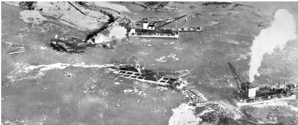
Figure 1.69: An immersed caisson (in the middle of the picture) to close a breach in the sea dike near Vlissingen, Zeeland (RAF, 1944)
