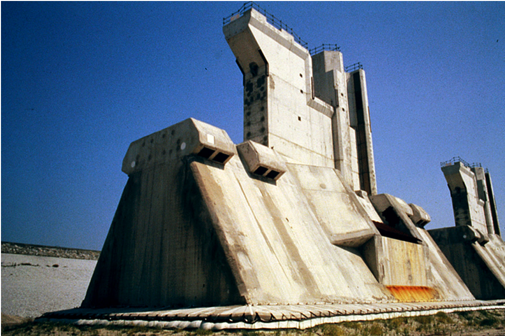
Figure 1.43: Precast pier for the Oosterschelde Storm Surge Barrier in the construction dock (Beeldbank RWS)
