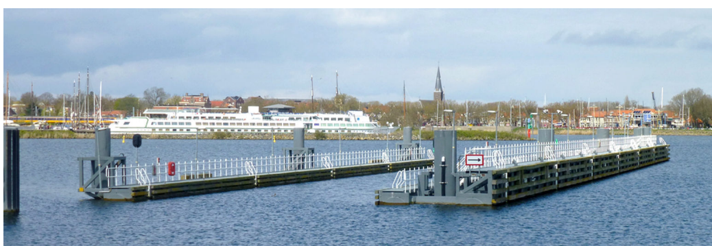
Figure 1.18: Berthing structure near the Naviduct of Enkhuizen (TU Delft, 2015)
