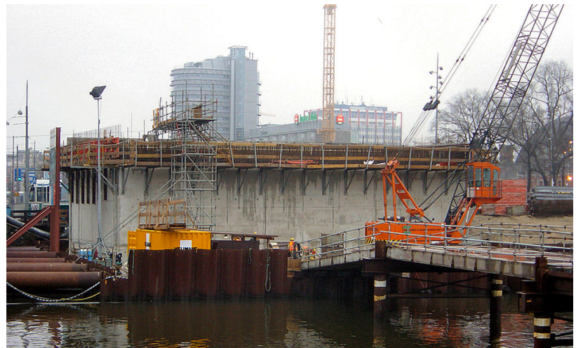
Figure 1.51: Schematic cross-section of a pneumatic caisson (left) and a picture of such a caisson before subsiding (right; Amsterdam – picture: TU Delft, 2008)
