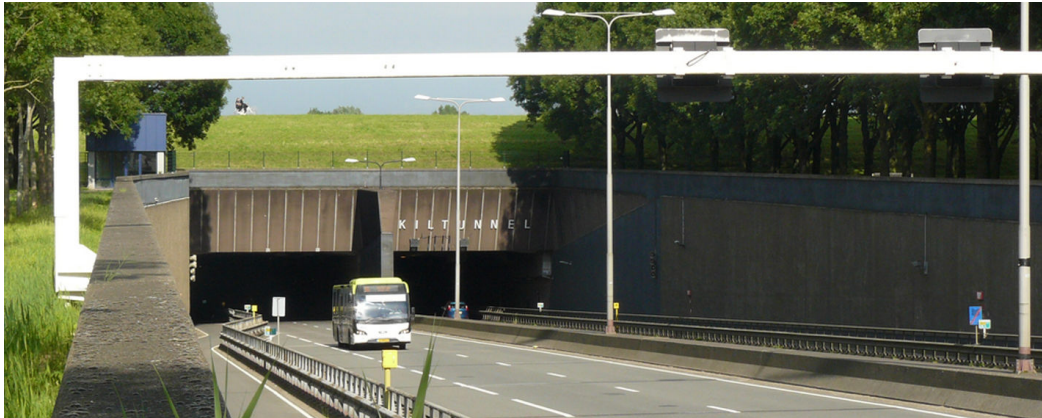
Figure 1.62: Approach to the Kiltunnel, Dordrecht (Wikimedia Commons, 2016)
