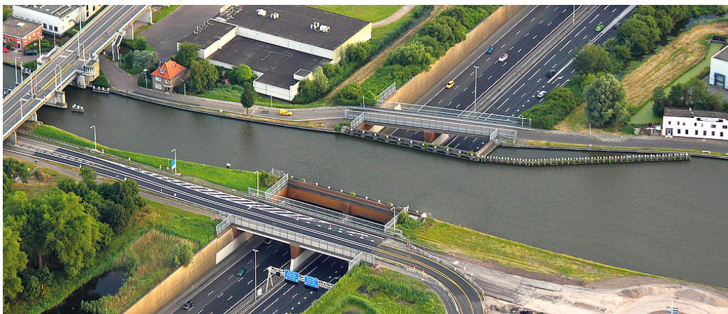
Figure 1.52: Gouwe aqueduct (RSK1992, flickr.com)
