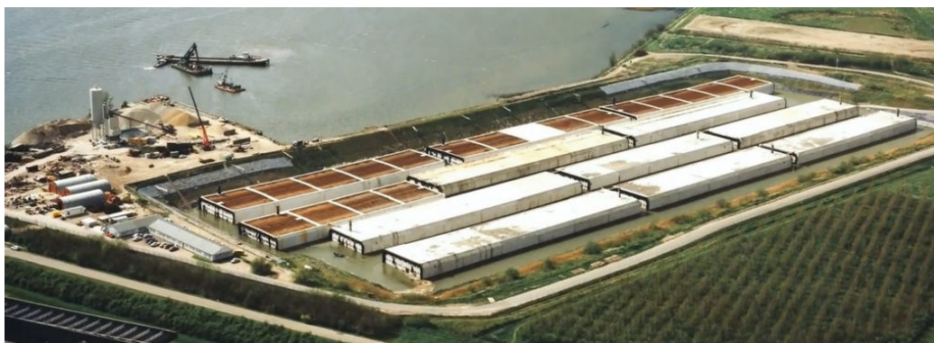
Figure 1.61: Tunnel elements in the construction dock near Barendrecht (Bas Romeijn, 2018)
