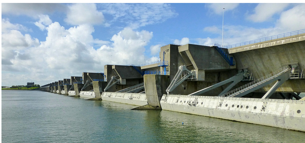
Figure 1.35: Haringvliet discharge sluices (TU Delft, 2014)
