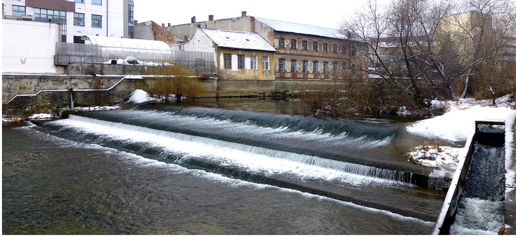
Figure 1.7: Fixed weir in the Someșul Mic in Cluj Napoca, Romania (TU Delft, 2013)
