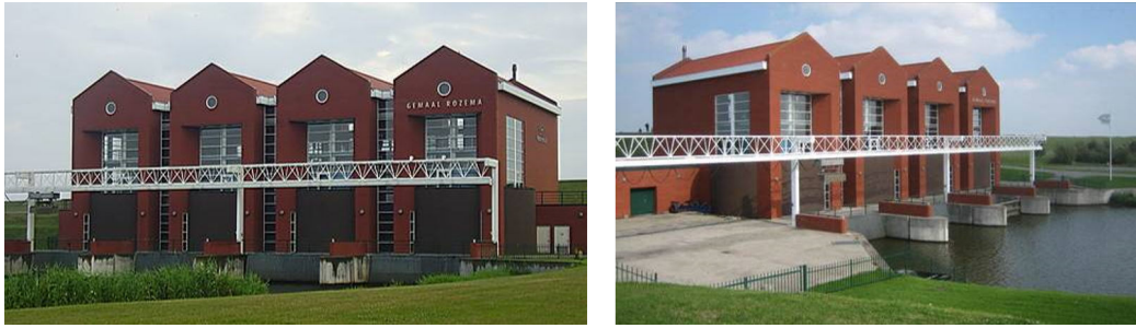
Figure 1.32: Pumping station Rozema near Termonterzijl
