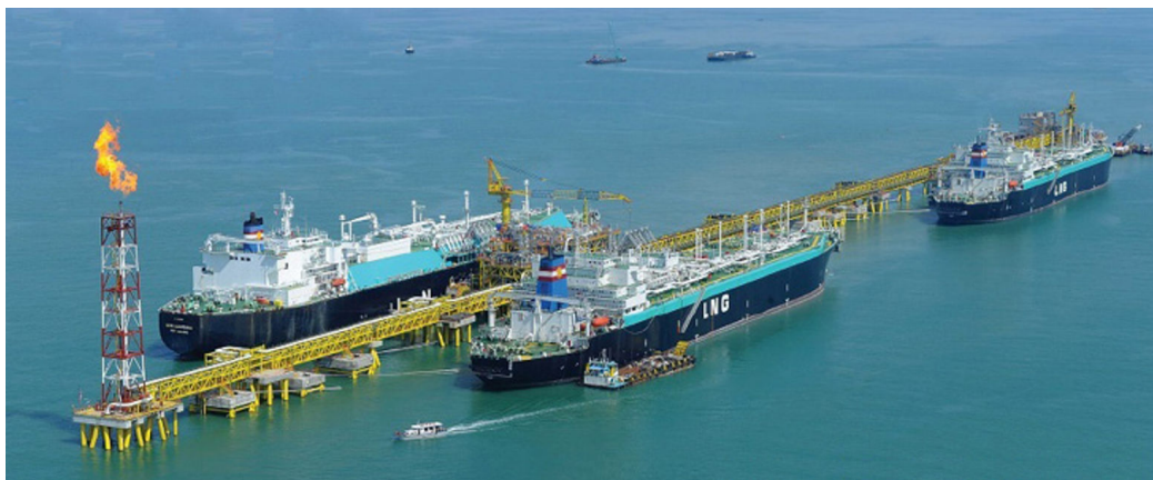
Figure 1.17: Detached jetty in Malaysia ( http://www.citech.co.uk )
