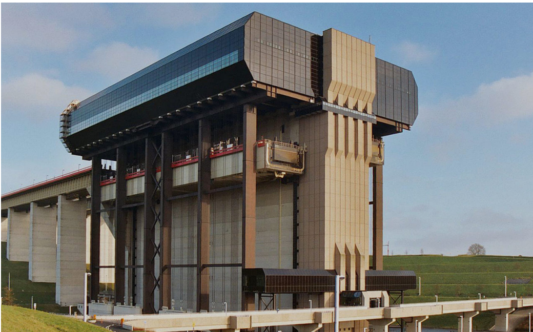
Figure 1.6: Cable ship lift of Strépy-Thieu, Belgium, with a vertical lift of 75 m (Wikimedia Commons, 2005)
