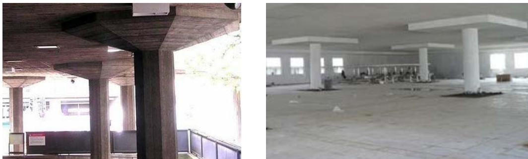
Fig. 14. 4: Flat slabs with a) column heads and b) drop panels
