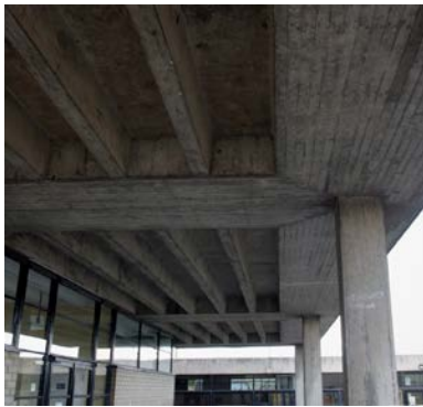
Fig. 14. 5: a) Ribbed and b) waffle slabs
