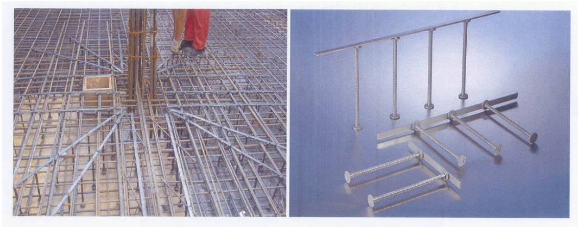
Fig. 14. 97: Applying shear studs as punching shear reinforcement
