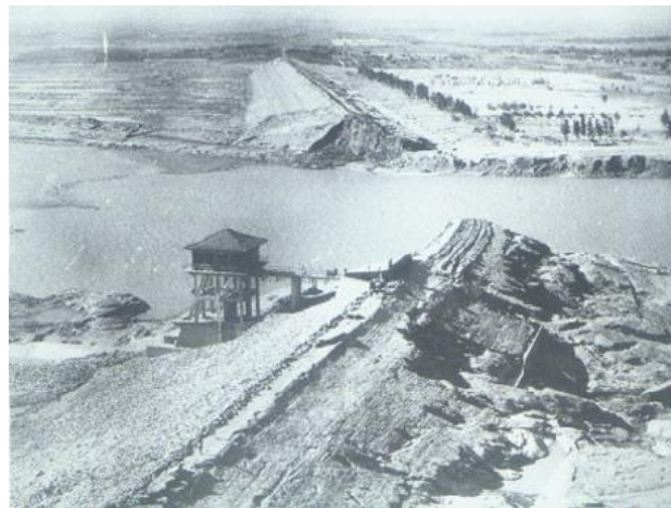
Figure 10.11 The Banqiao dam after failure due to heavy rain (Sharpe, 1998)
